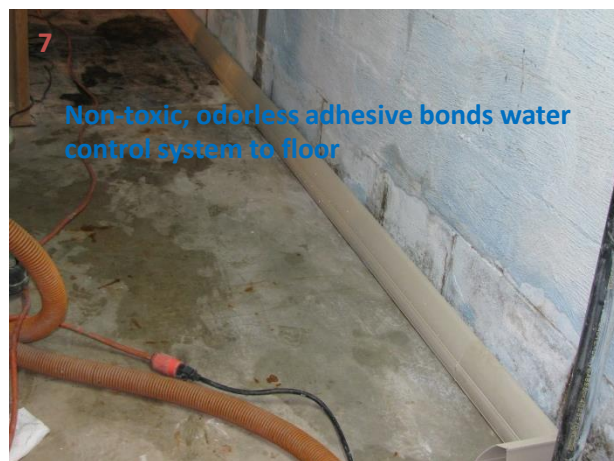
Water drains from holes & floor is prepared for system installation
