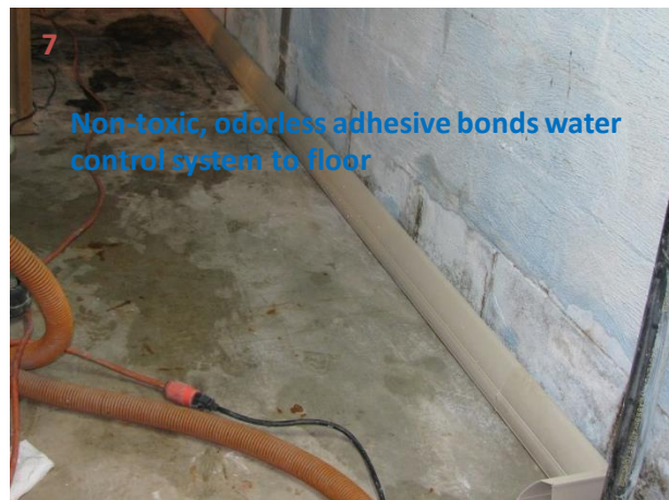
Sections are connected with waterproof couplings
